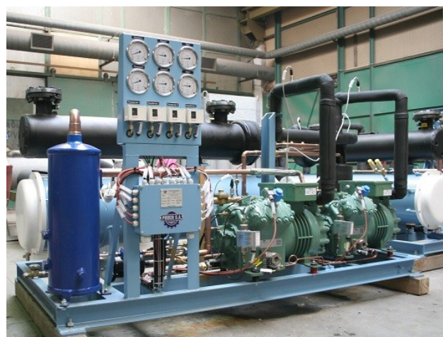
Chiller for air-conditioning system on Zodiak II
